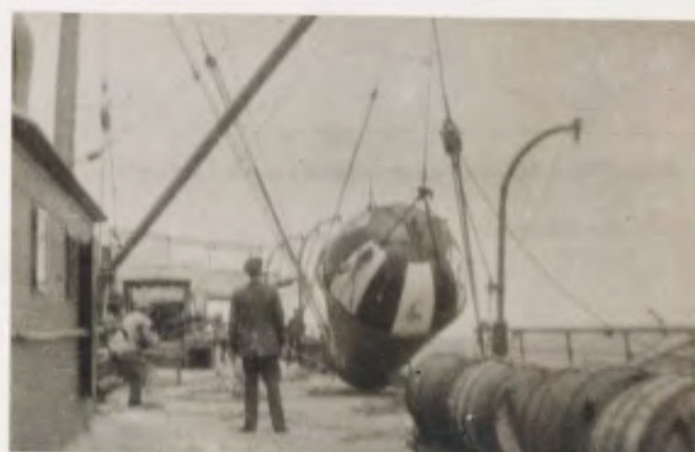
4. Lowering a buoy on deck.
