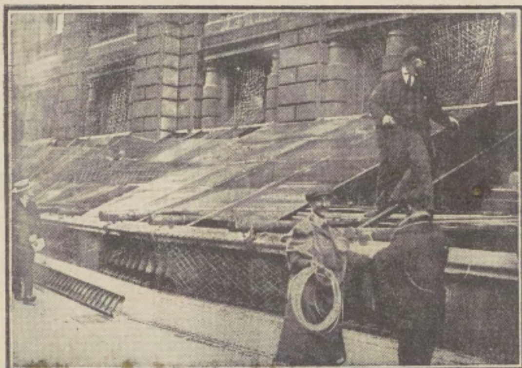
The Government are taking every precaution to safeguard telegraphic communication against bomb throwers by placing torpedo netting over the most important offices.
