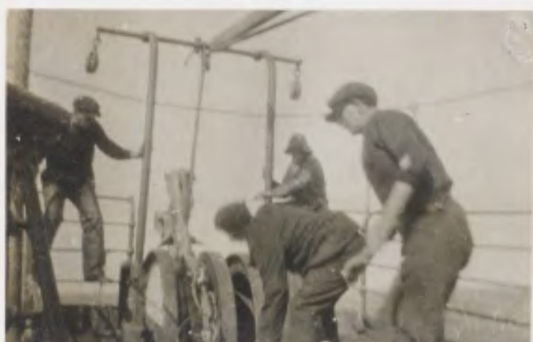
3. Getting a Lucas cutting Grapnel on board.
